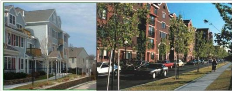
Transit Oriented Design district will use Chapter 40R provisions to allow for expanded higher density housing opportunities.
