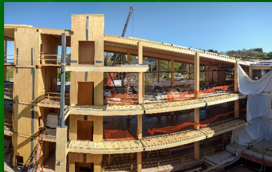
Olver Design Building - UMass
